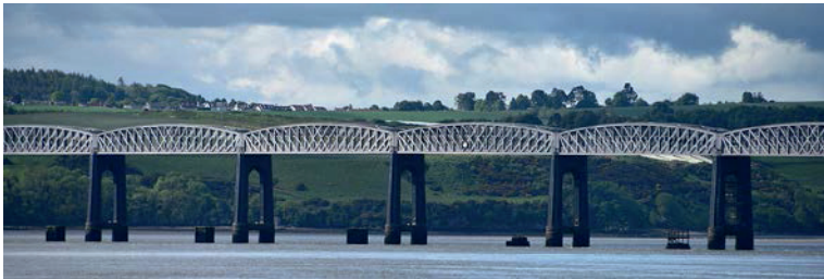
Northern segment of the second Tay Bridge, showing stumps of the original bridge's piers poking above the Tay
